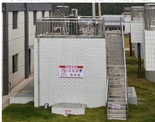
污泥调理池加盖
