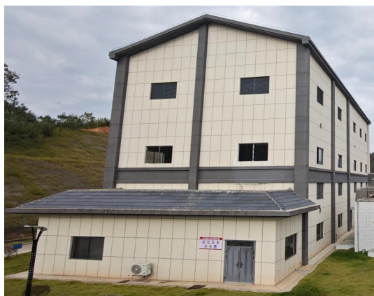
污泥脱水车间密闭
