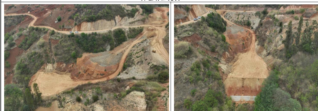
弃渣场区现状
