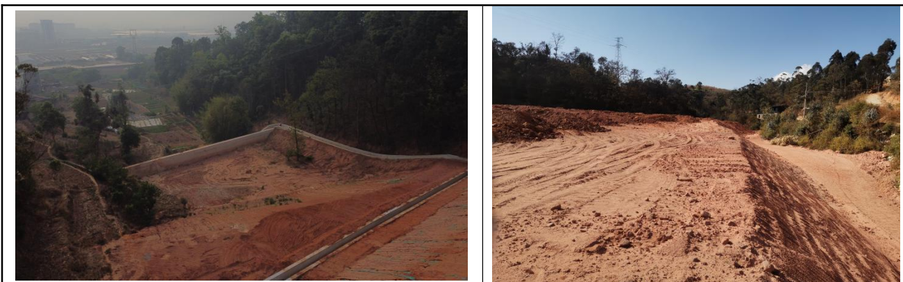
弃渣场区现状
