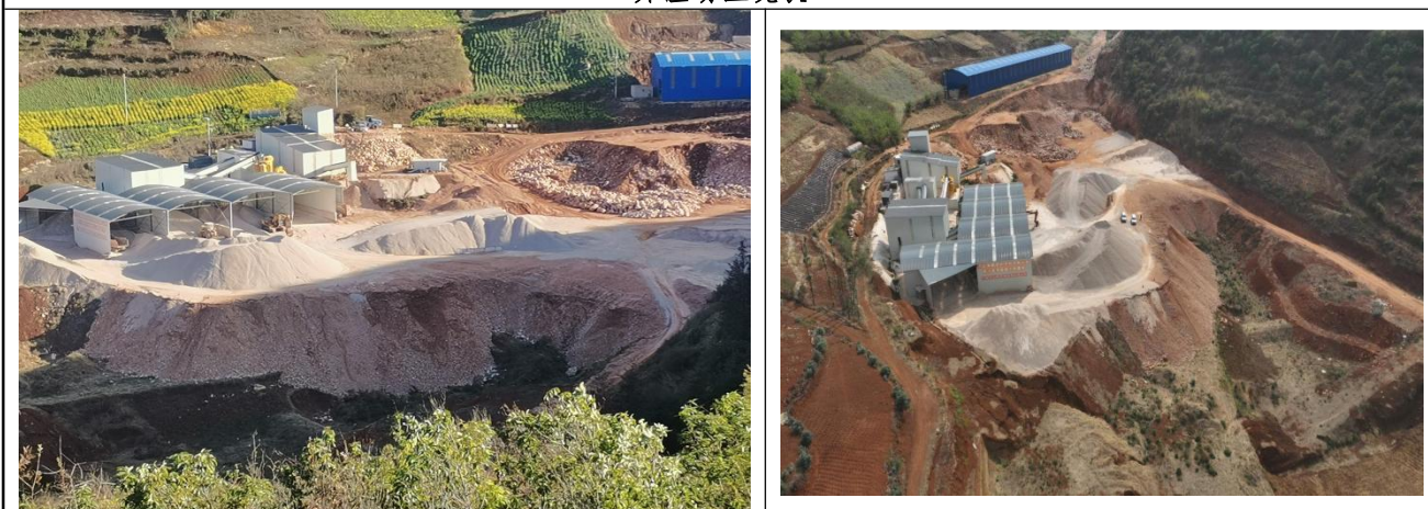
弃渣场区现状
